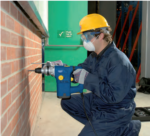
Figure 10.9 Electric drill with percussion hammer action to drill holes in masonry
