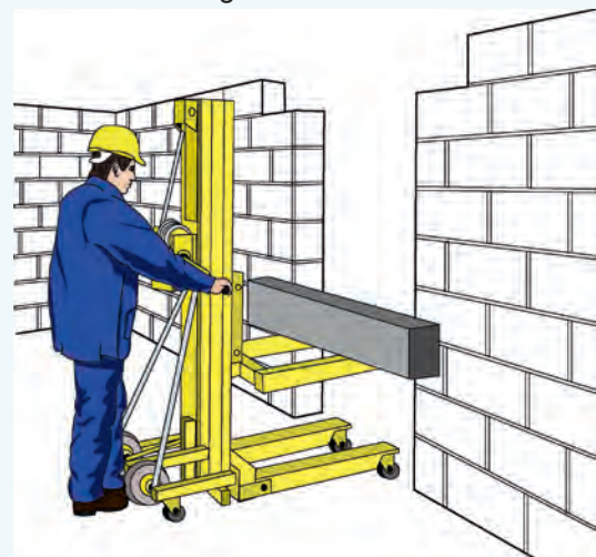
Use of hand-operated lift truck to place lintels
