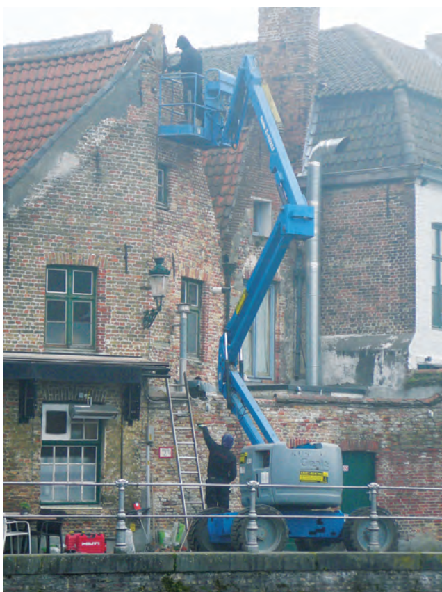
Figure 16.7 Good quality access on a MEWP for pointing brickwork in Belgium
