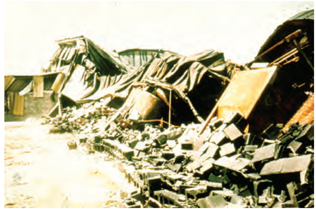
Figure 12.15 Steel structures can collapse in the heat of a fire
