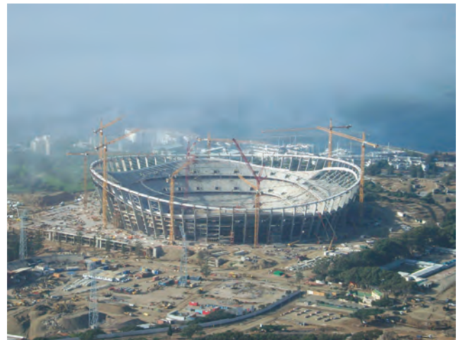
Figure 16.6 World Cup stadium, under construction, Cape Town, 2009
