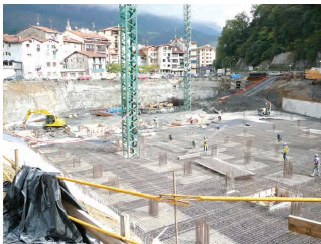
Figure 7.20 Groundwork clearance and foundations
