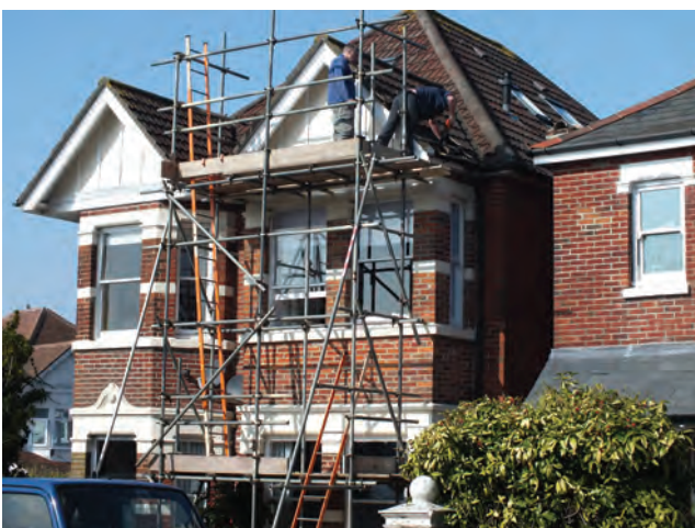
Figure 1.14 Domestic client: CDM applies but not notifiable because a short duration project
