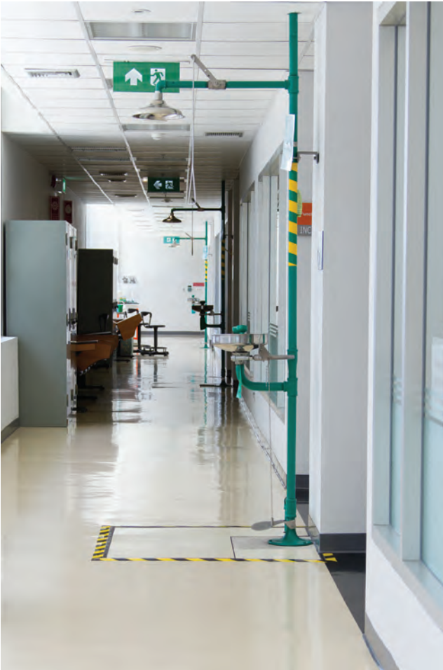
Figure 4.18 Emergency shower and eye wash station where there is a serious risk of chemical contamination
