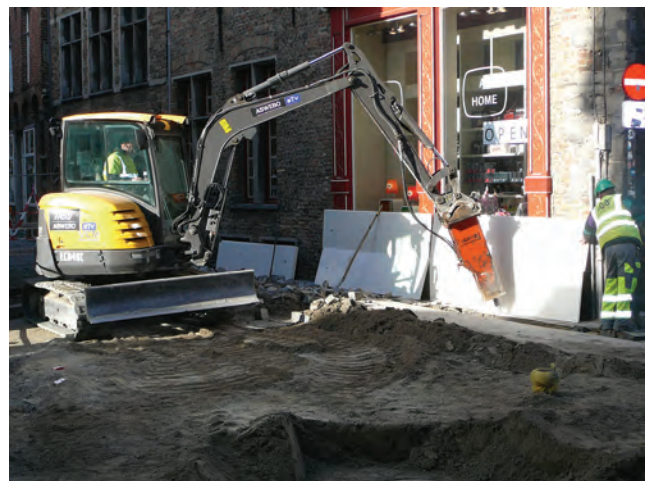
Figure 14.6 Breaker mounted on an excavator's jib to reduce vibrations
