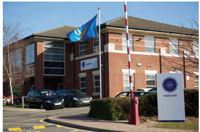
Figure 1.9 NEBOSH is in control here
