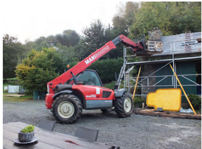
Figure 9.1 Handling roofing slates onto a roof using a teleporter lift truck
