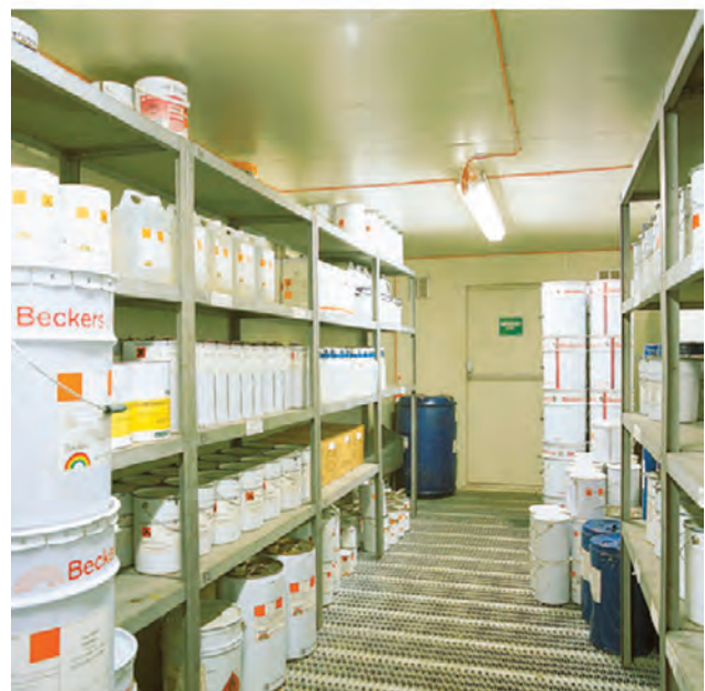
Figure 12.14 Various storage arrangements for highly flammable liquids
