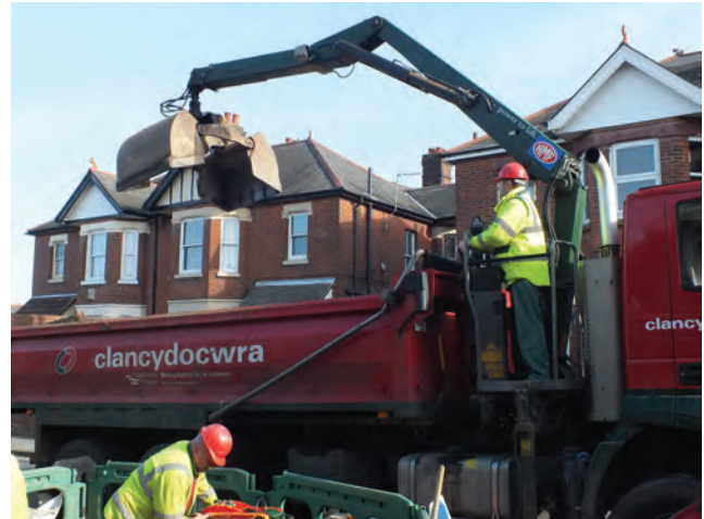
Figure 1.16 Contractors at work using a lorry-mounted loading grab
