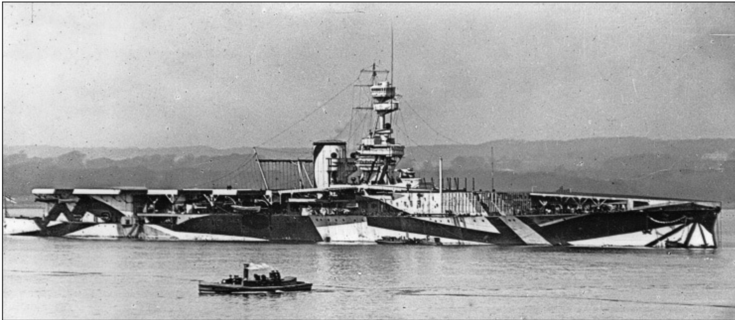
Furious in a disruptive pattern paint scheme in 1918, after modification with a landing-on deck aft. Note the prominent 'goal post' and rope barrier intended to prevent aircraft from crashing into the funnel. (AUTHOR'S COLLECTION)
