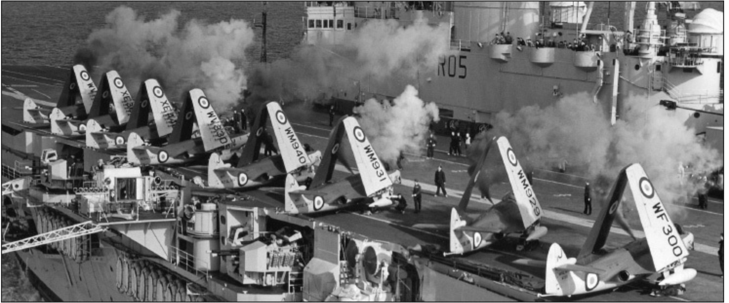
Sea Hawks starting up together in Eagle ; the smoke is the exhaust from their cartridge starter units. (AUTHOR'S COLLECTION)
