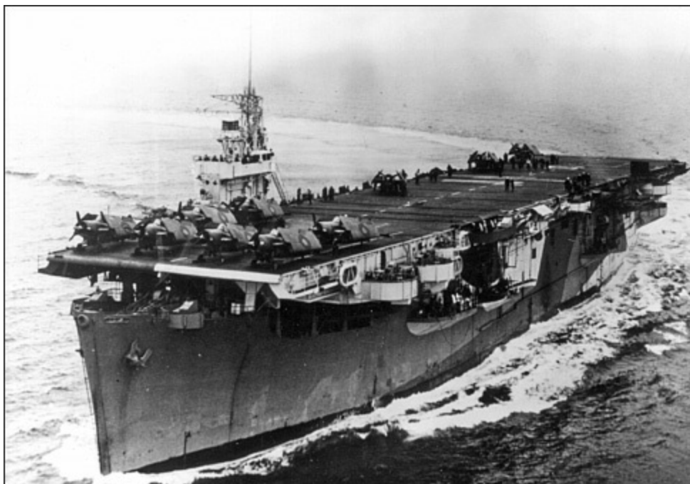
Searcher turns out of wind after landing-on a number of 882 NAs Wildcats. Handling teams have started to move aircraft aft out of Fly 1 into the range aft. (AUTHOR'S COLLECTION)
