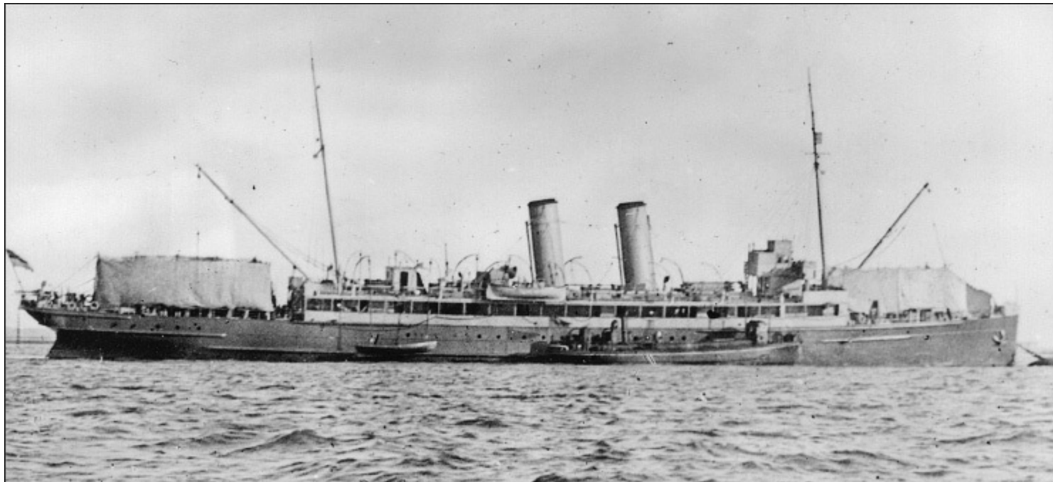
Riviera in 1914, shortly after her initial conversion, with canvas hangars and derricks fitted in Chatham Dockyard. (AUTHOR'S COLLECTION)
