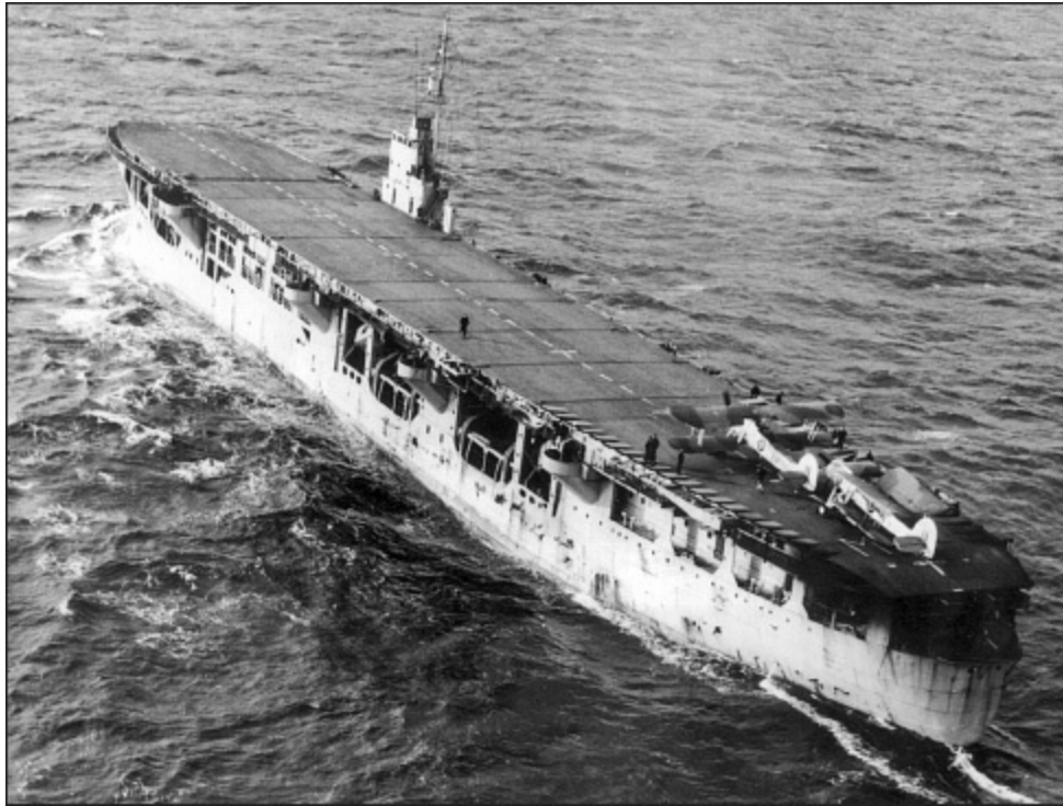
The ‘tanker’ MAC-Ship Amastra with two of her Swordfish ranged aft and windbreaks down. (AUTHOR'S COLLECTION)
