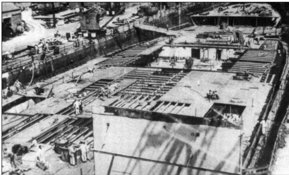
Victorious in dry dock early in her reconstruction, showing the extent to which she was cut down before being rebuilt. (AUTHOR'S COLLECTION)
