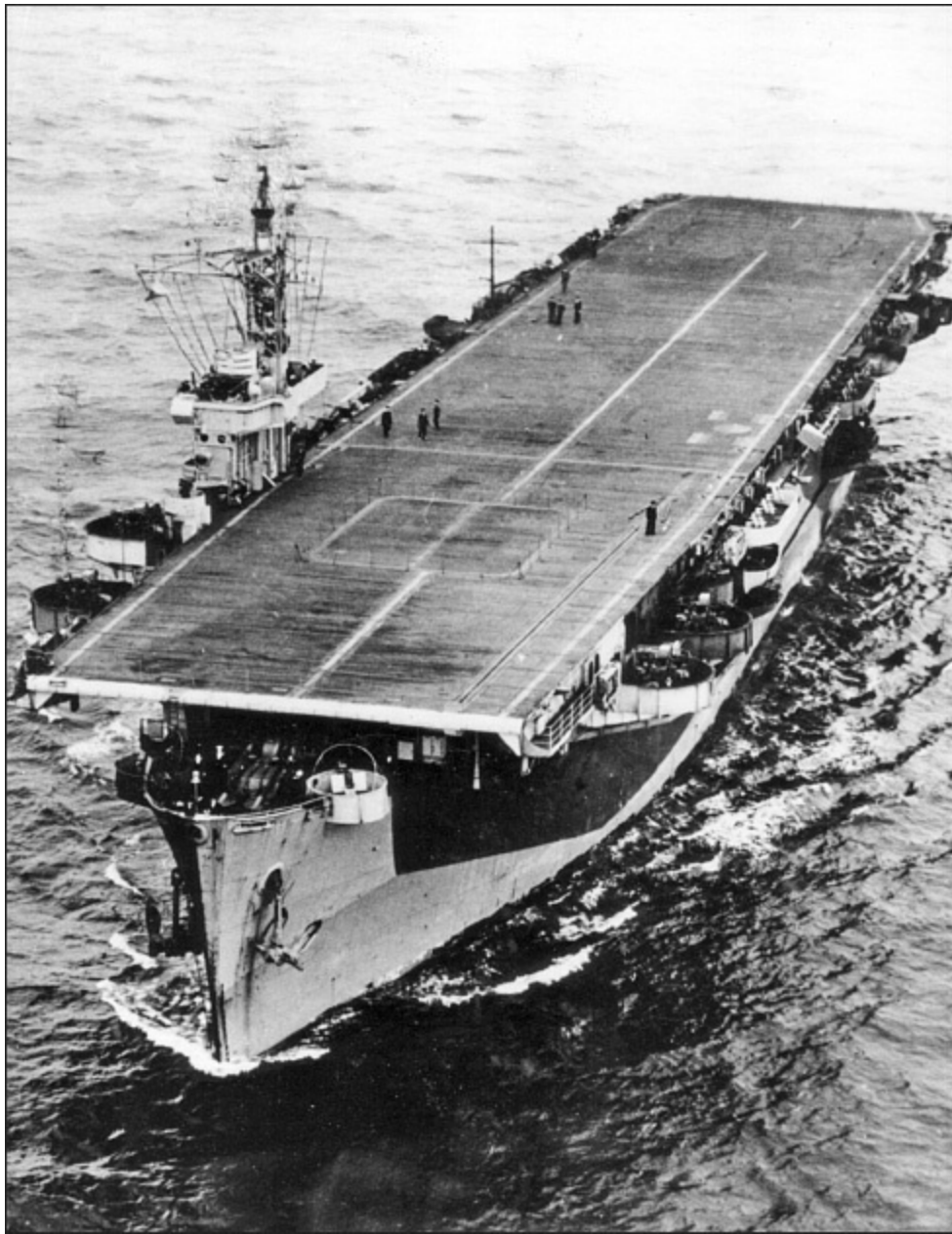
Queen , clearly showing her aircraft signal panels on the port side of the flight deck amidships. (AUTHOR'S COLLECTION)
