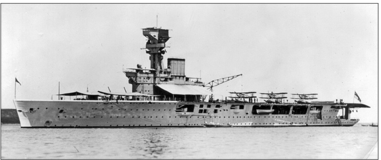
Anchored off Wei-Hei-Wei on the China Station, Hermes is seen operating Fairey IIF seaplanes from her flight deck. The crane is about to lift the forward aircraft on to the water. Awnings have been spread over part of the flight deck to protect men working. The concept of operating seaplanes from a carrier at anchor was not finally discarded until 1940. (AUTHOR'S COLLECTION)
