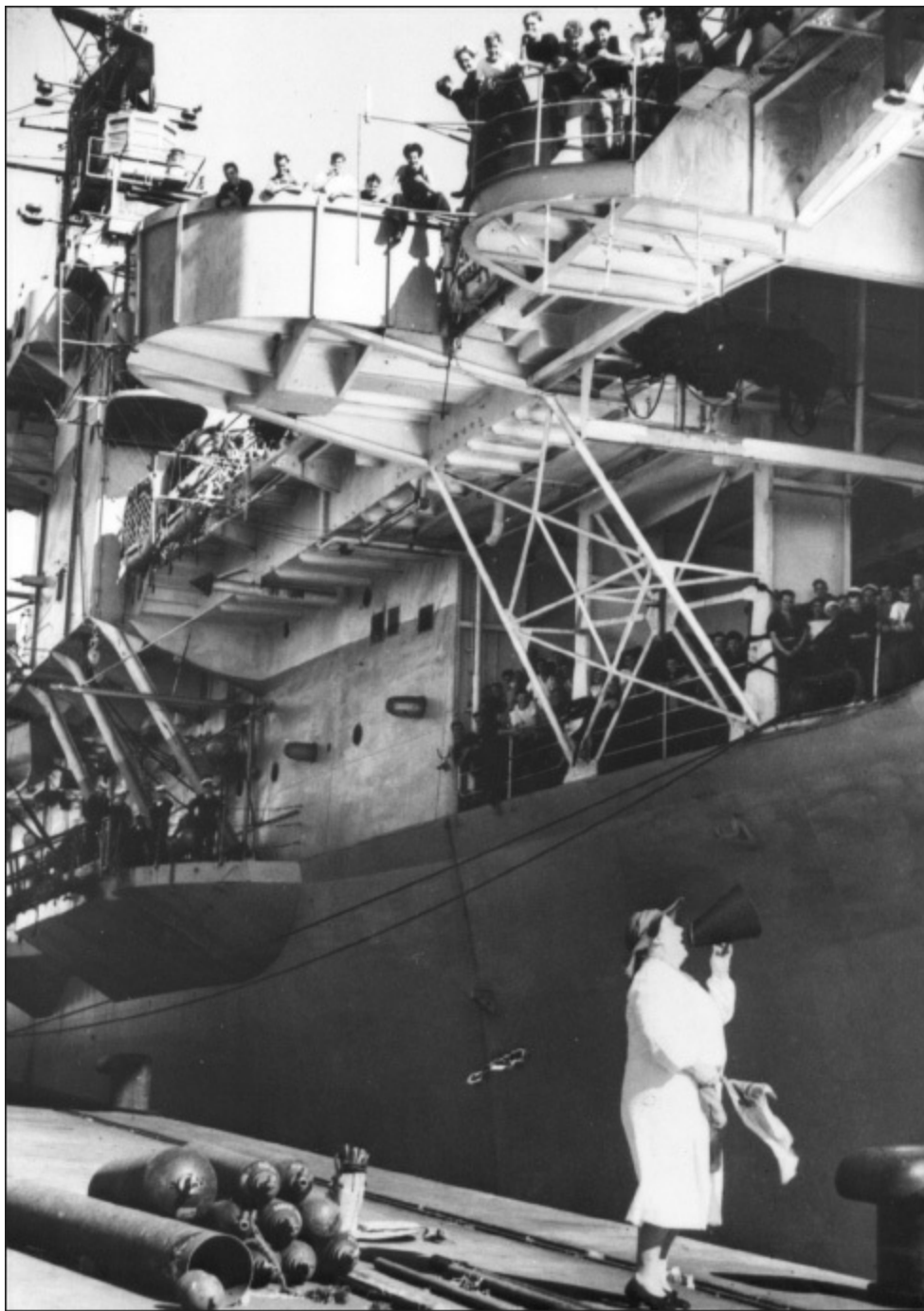
The ‘White Lady’ singing for Battler in Durban in 1944. The photograph gives a good view of the structure that supported the starboard sponsons. (AUTHOR’S COLLECTION)
