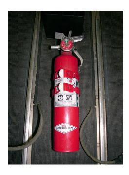
(approximately 125 psi) and the operating lever lock pin is securely in place.
