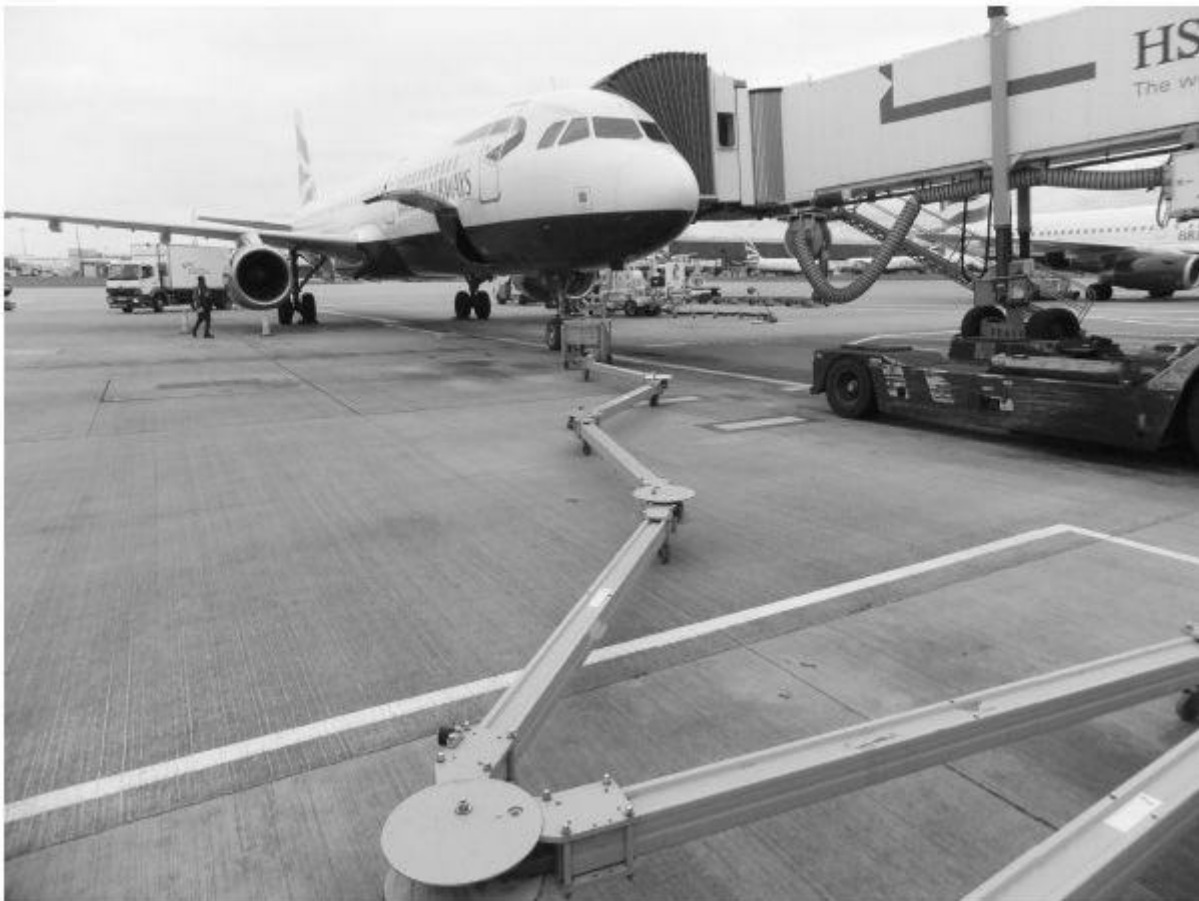
FIGURE 6.13 Apron cable electrical supply.
