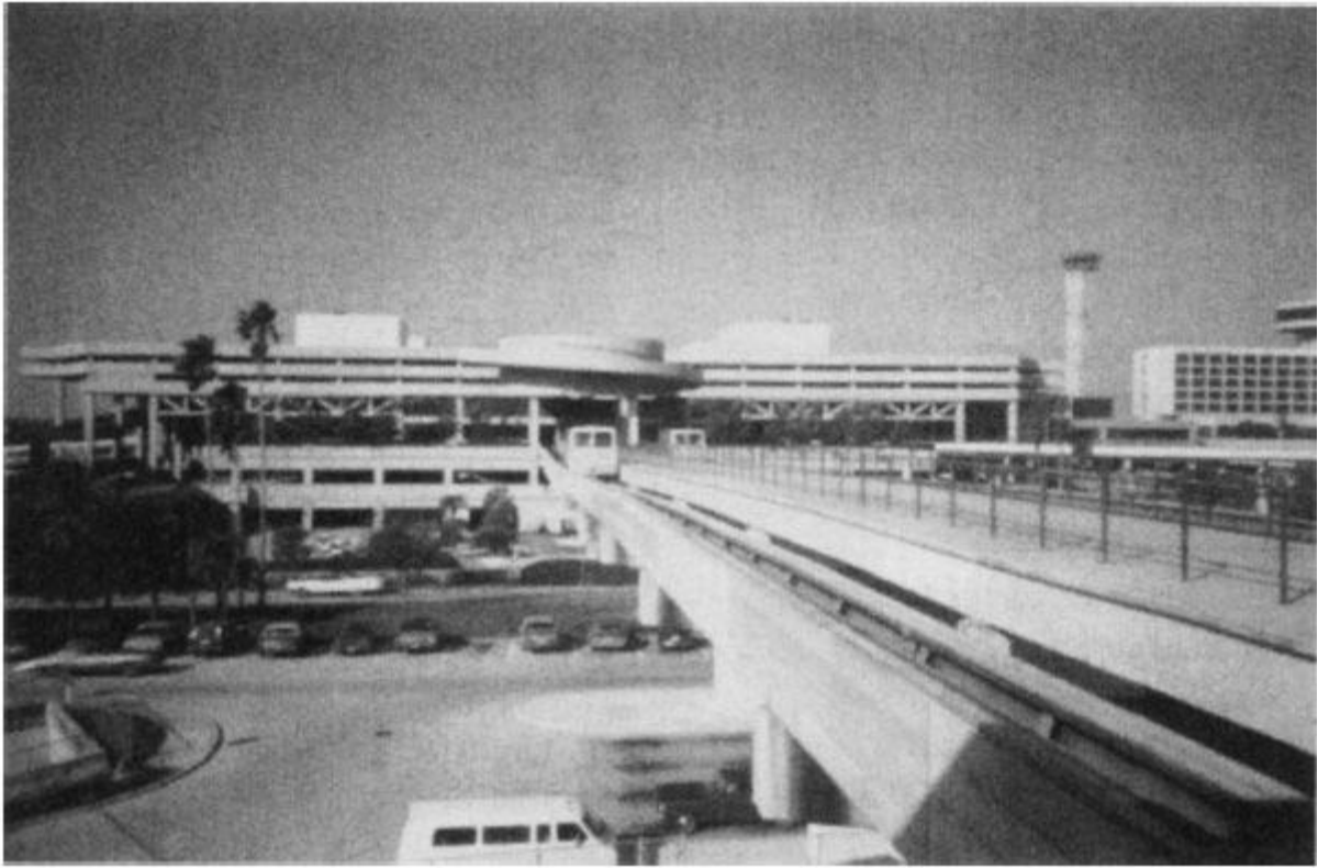
FIGURE 8.26 People mover on track between main terminal and satellite at Tampa International Airport.
