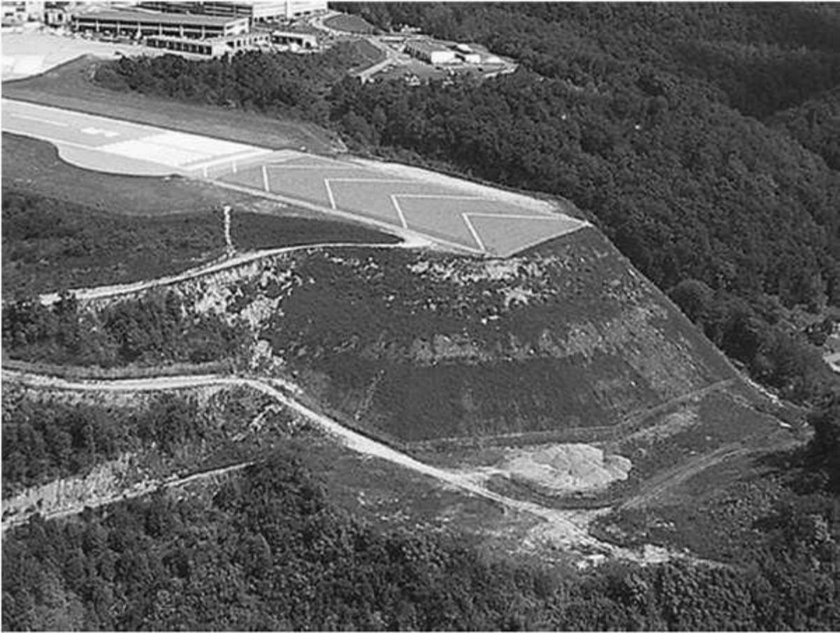
FIGURE 11.3 EMAS installation at Charleston Airport, West Virginia. (Source: Charleston Airport.)
