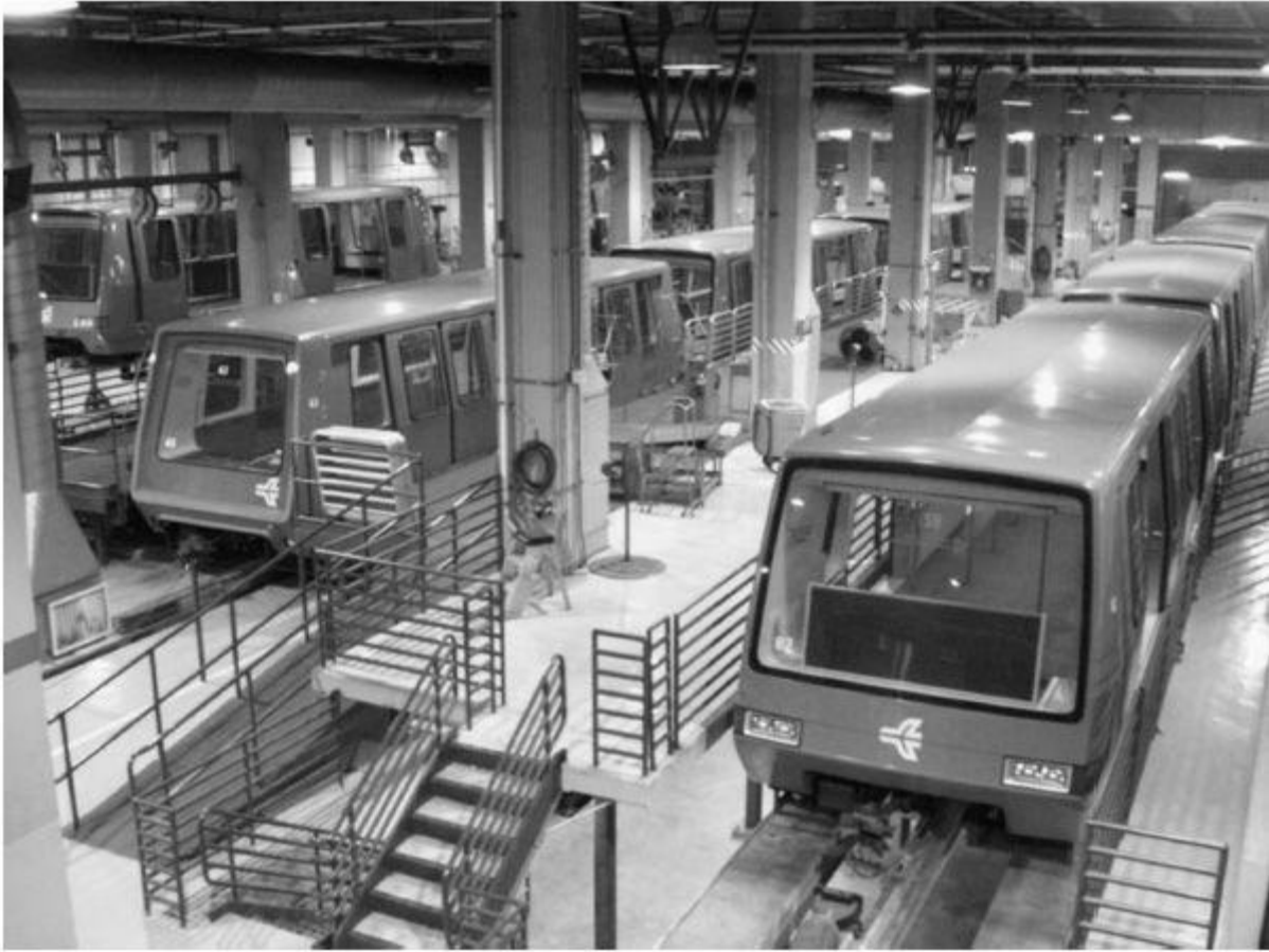
FIGURE 8.28 People mover in maintenance area. (Note the pit for maintenance under the rails.)
