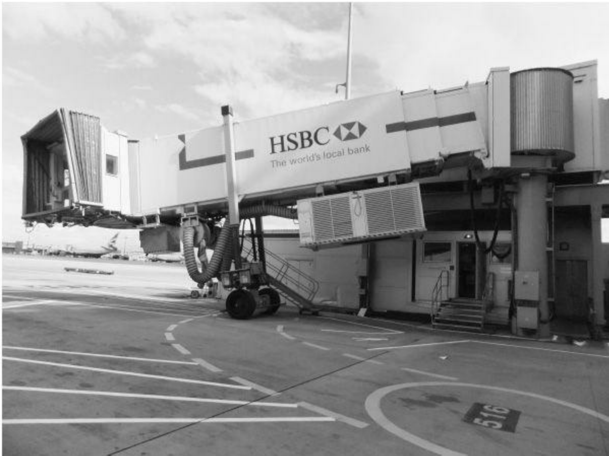
FIGURE 6.15 Fixed ground cooling unit attached to an air bridge.
