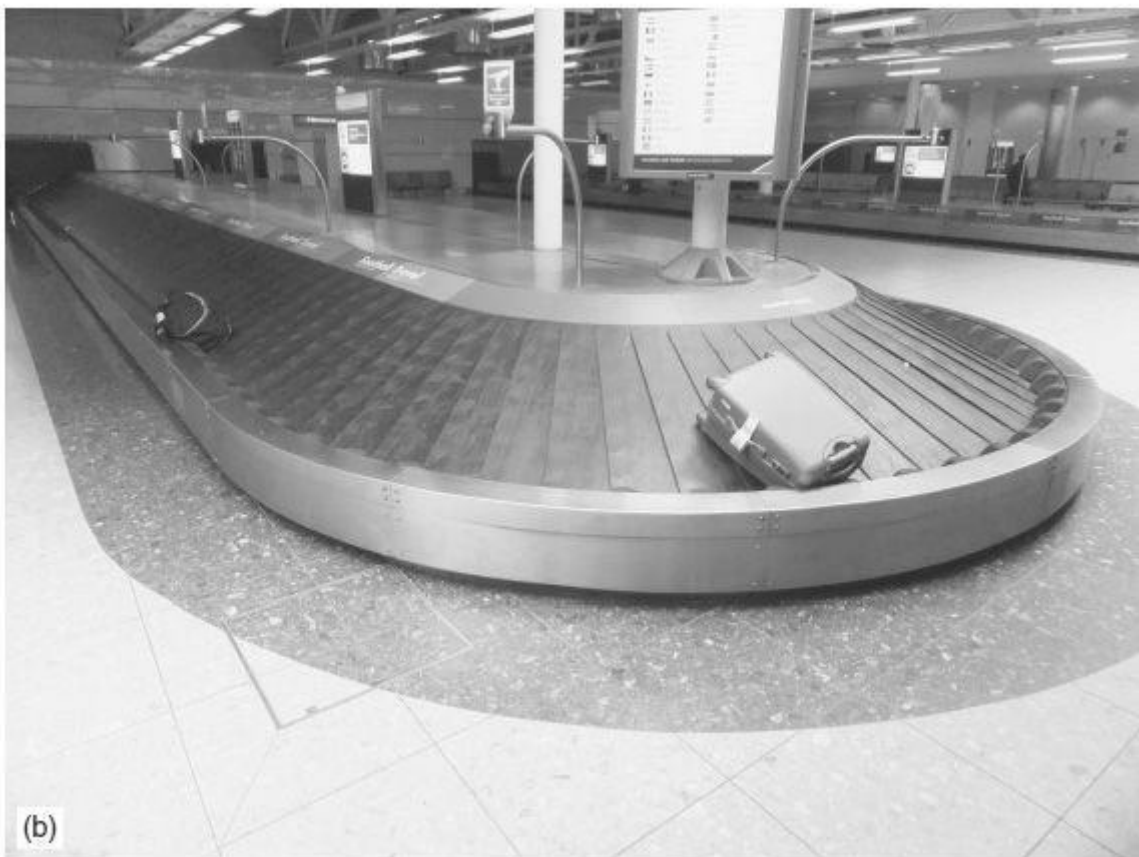
FIGURE 7.18 (a) Flatbed reclaim. (b) Inclined reclaim.
