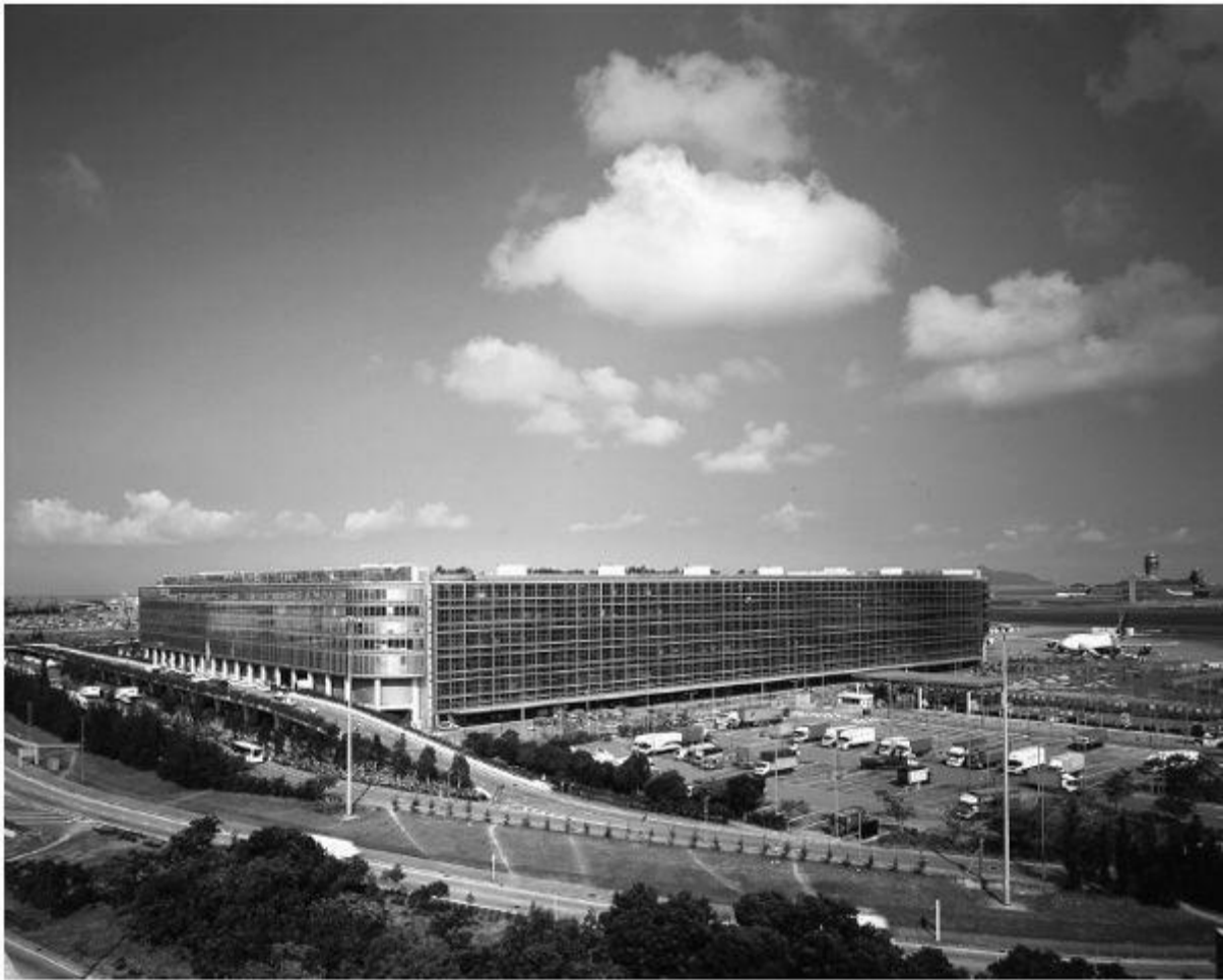
FIGURE 10.13 HACTL Terminal, Hong Kong. (Courtesy: Hong Kong International Airport.)
