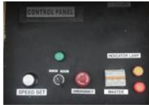
6. Control Panel Wind Tunnel
