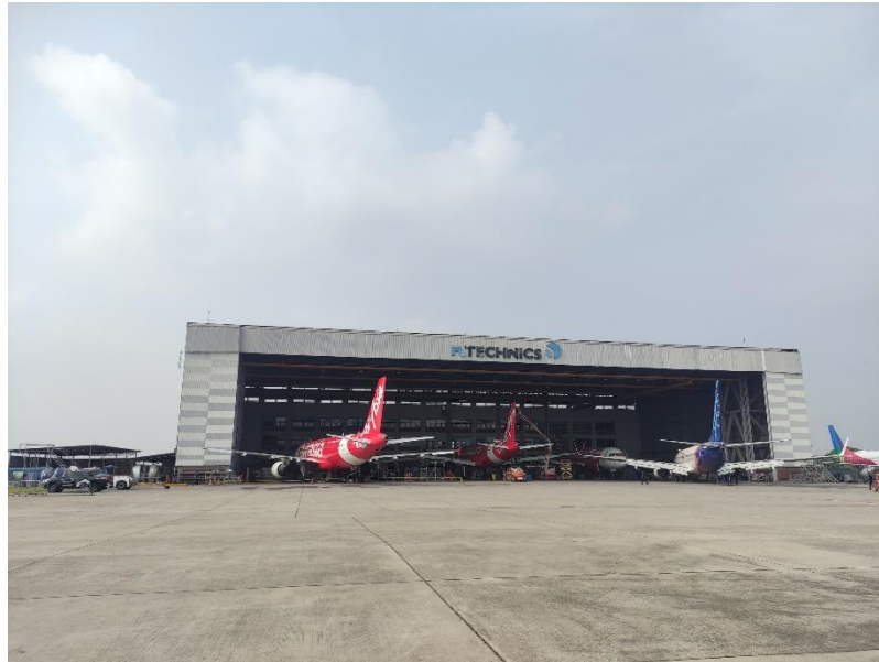
Gambar 2.1 Hangar FL TECHNIC INDONESIA - Cengkareng
