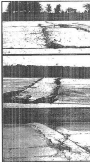
Gambar 3. 1 Retak Hancur (Blow Up)
