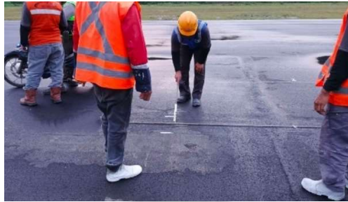
Gambar 4. 21 Contoh Proses Premarking Runway Centre Line Marking (Sumber: Dokumentasi Pribadi, 2024)
