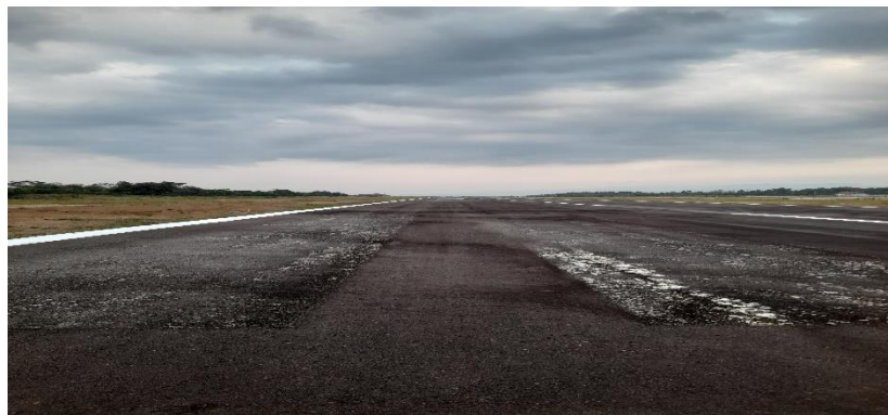
Gambar 4.24 Marka Touchdown Zone Sebelum Proses Pengecatan
