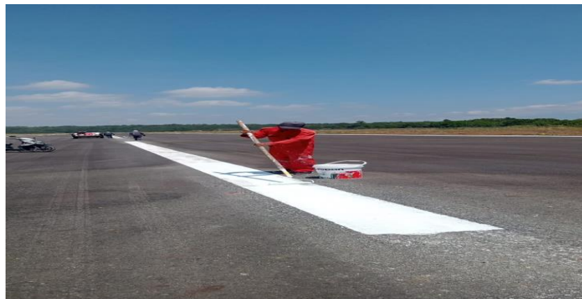
Gambar 4.22 Proses Pengecatan Marka Center Line
