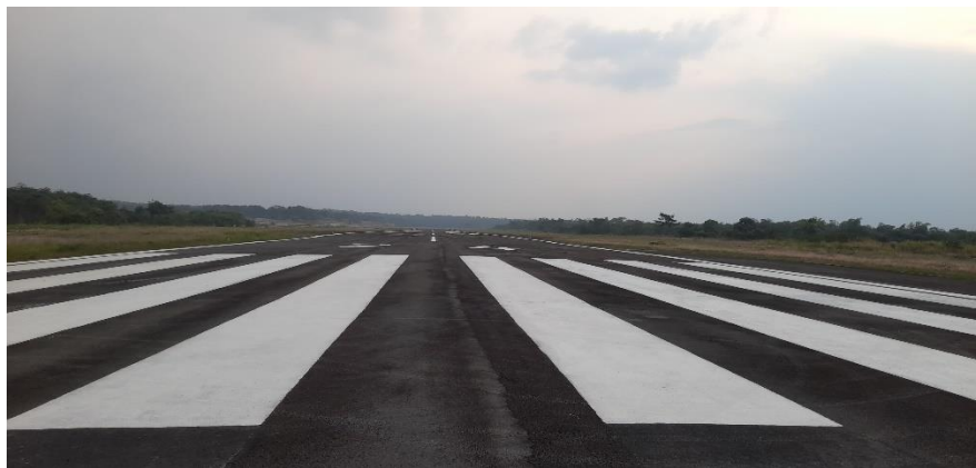
Gambar 4.21 Hasil Pengecatan Marka Threshold
