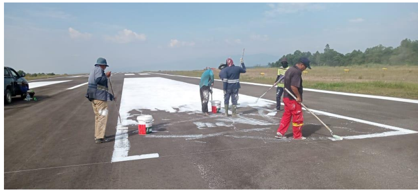
Gambar 4.18 Proses Pengecatan Marka Aiming Point
