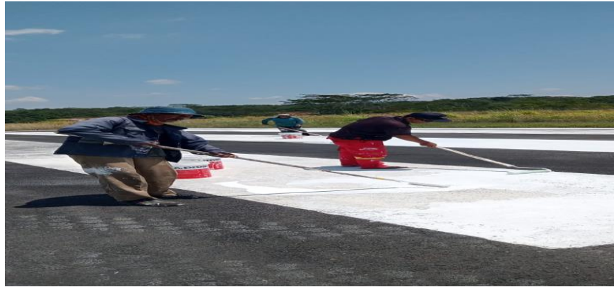
Gambar 4.20 Proses Pengecatan Marka Threshold
