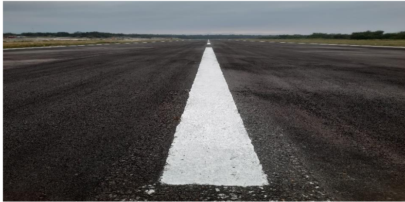
Gambar 4.23 Hasil Pengecatan Marka Center Line
