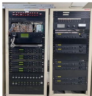
Gambar 3 . 13 Rack Public Address System
