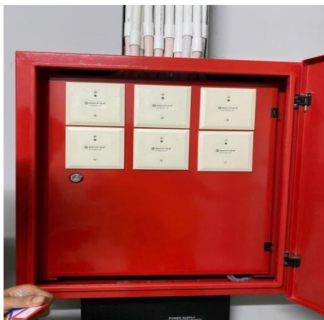
Gambar 3 . 14 Junction Box Fire Alarm
