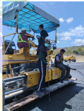
Penghamparan Aspal AC-BC di area perpanjangan runway
