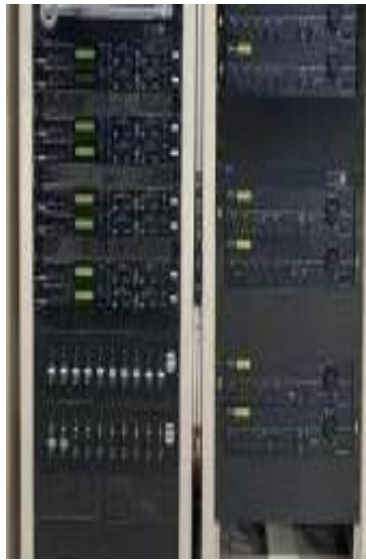
Gambar 3 . 9 Rack Public Address System
