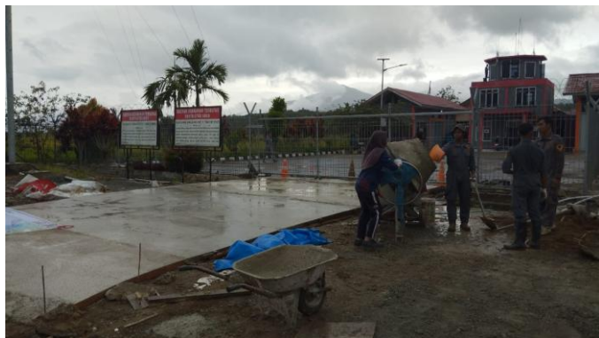
Gambar 4. 106 Penegcoran Beton
