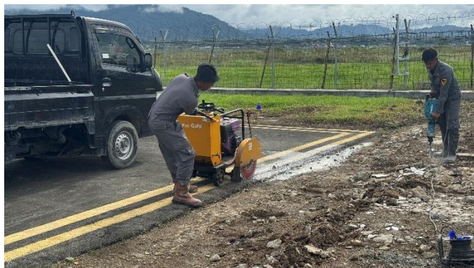
Gambar 4. 96 Cutting Asphalt
