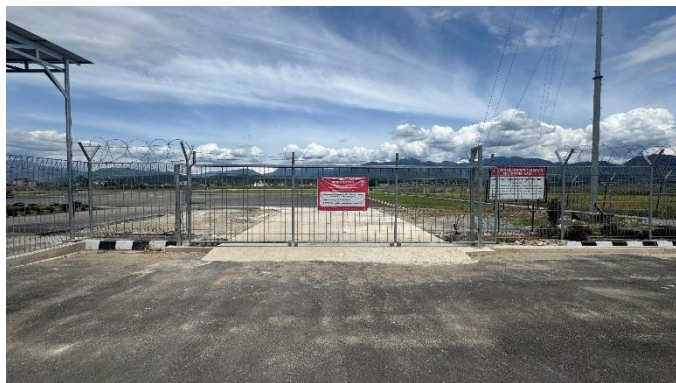
Gambar 3. 40 Jalan Akses Masuk Airside
