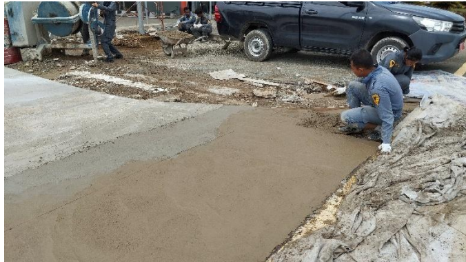
Gambar 4. 107 Finishing Beton
