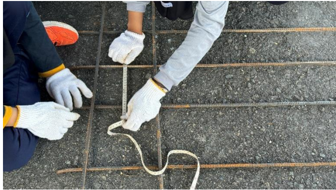
Gambar 4. 99 Pengukuran Wiremesh
