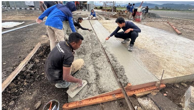
Gambar 4. 105 Perataan Beton
