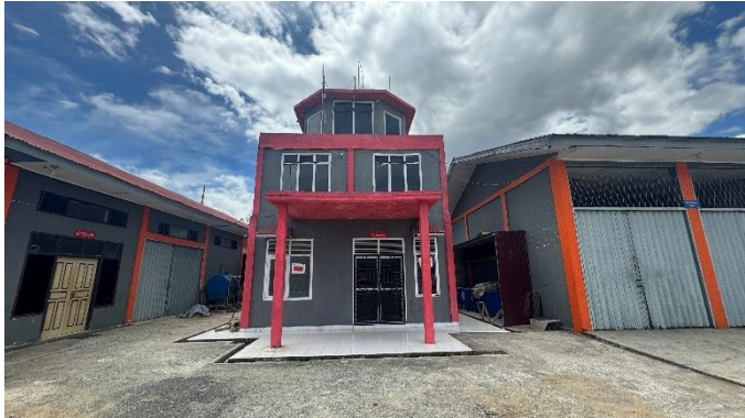
Gambar 4. 10 Gedung Menara Airnav (Tower)
