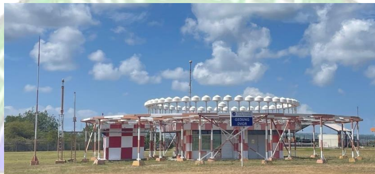
Gambar 3. 16 Ground Station DVOR
