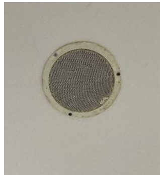
Gambar 3. 9 Ceiling Speaker Public Address System
