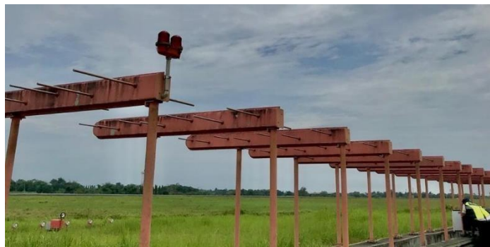
Gambar 3 . 11 Antenna Localizer 03
