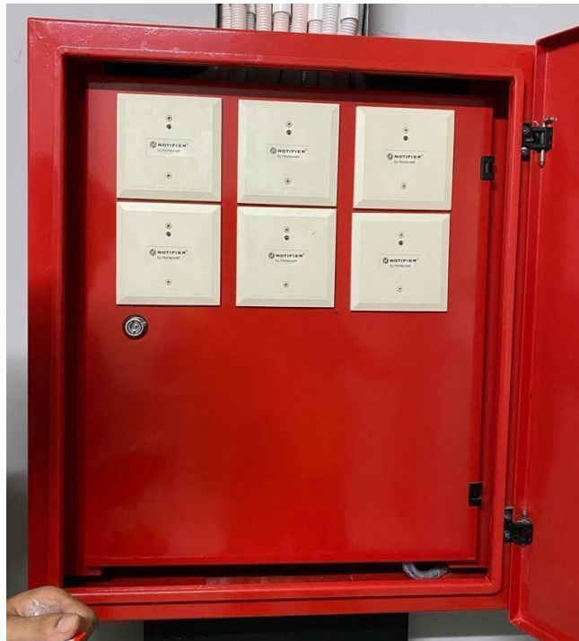
Gambar 3 12 Junction Box Fire Alarm
