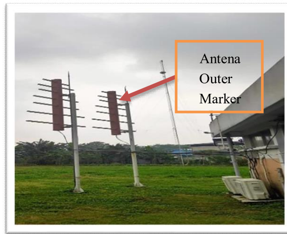
Gambar3. 17 Antena Outer Marker 25R
