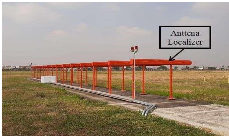
Gambar3. 15 Antena Localizer 25L
