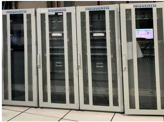
Gambar3. 10 Kabinet VCCS Frequentis
