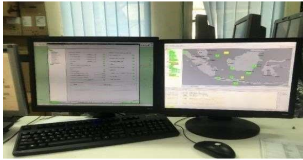
Gambar 3. 21 RCMS ADS-B Di Processing Room
