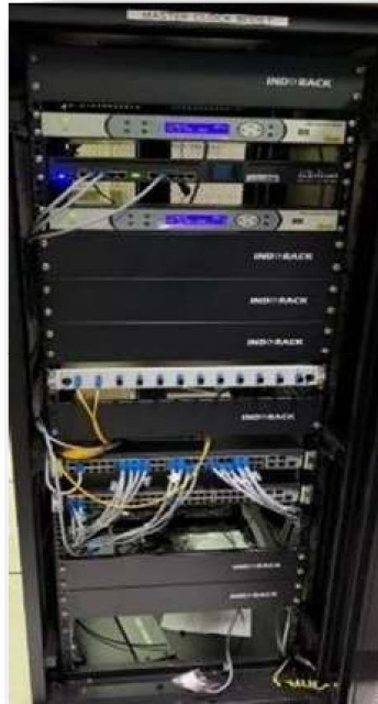
Gambar3. 14 Server NTP Master Clock
