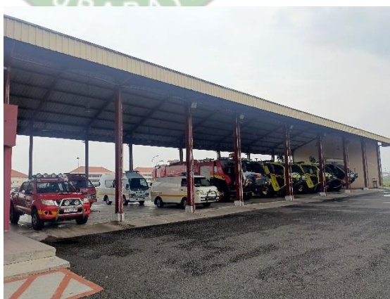
Gambar 4. 21 Gedung Fire Station Terminal 1
