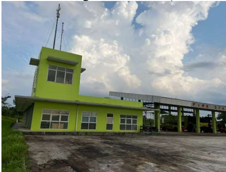
Gambar 4. 6 Bangunan PKP-PK (Fire Station)
