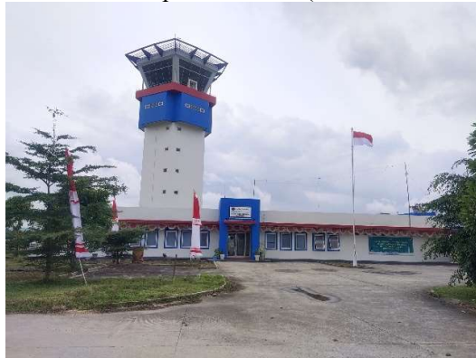
Gambar 4. 5 Kantor personel ATC (ATC Office Building)
