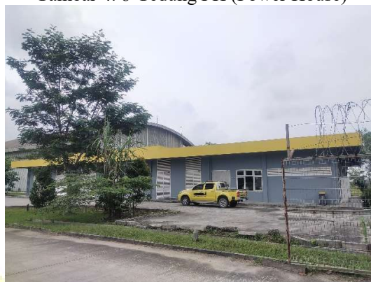
Gambar 4. 8 Gedung PH (Power House)
