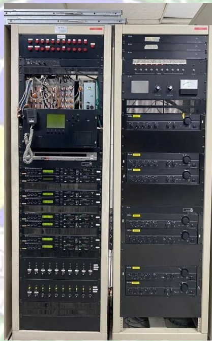
Gambar 3. 9 Rak Public Address System (PAS)
