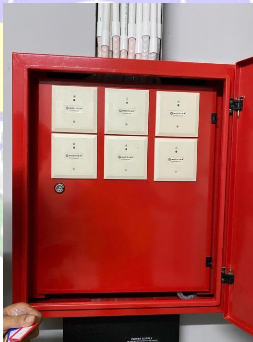
Gambar 3. 10 Junction Box Fire Alarm
