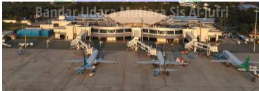
Gambar 2. 4 Apron Bandara Sumber : Website Bandara
