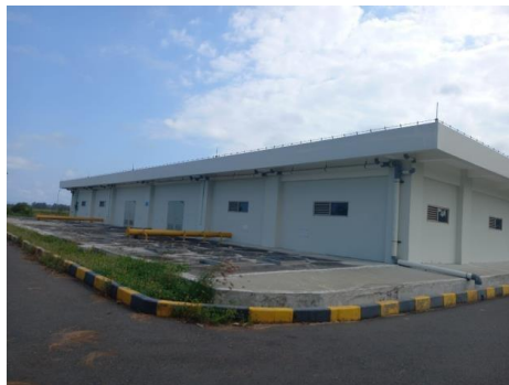
Gambar 4. 13 Sewage Treatment Plant (STP) (Sumber : Dokumentasi Penulis,2024)
