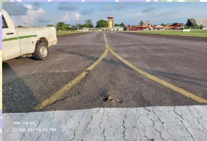
Gambar 4. 1 Kerusakan Rutting di Taxiway Alpha
