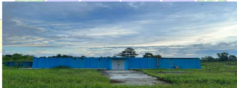
Gambar 4. 16 Water Treatment Plant (WTP)
