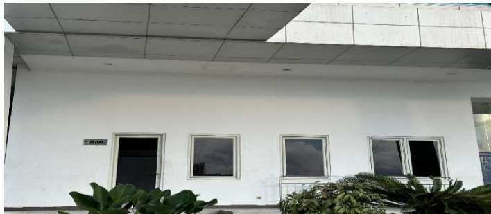
Gambar 4. 14 AMC Office (Apron Movement Control)
