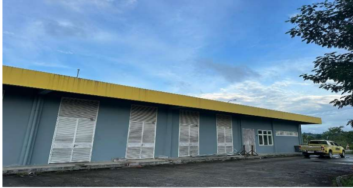
Gambar 4. 12 Gedung Power House
