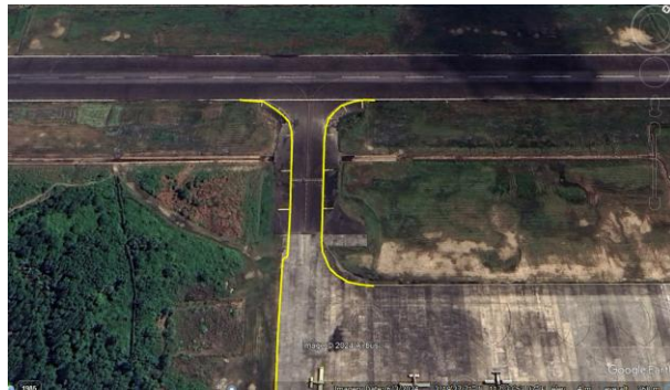
Gambar 4. 12 Taxiway C (Sumber : Google earth )
