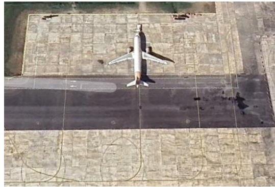
Gambar 4. 15 Lokasi perpindahan parking stand 1-6 ( West Apron ) (Sumber : Google earth )
