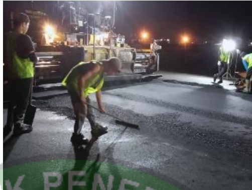
Gambar 4. 21 Meratakan hamparan asphalt join
