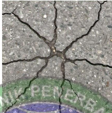
Gambar 3. 7 Map Cracking (Sumber : www.google.com 2024)
