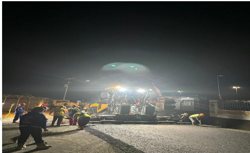
Gambar 4. 4 Trial Compaction
