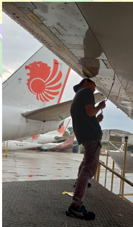
Gambar 4.42 Proses removal panel
