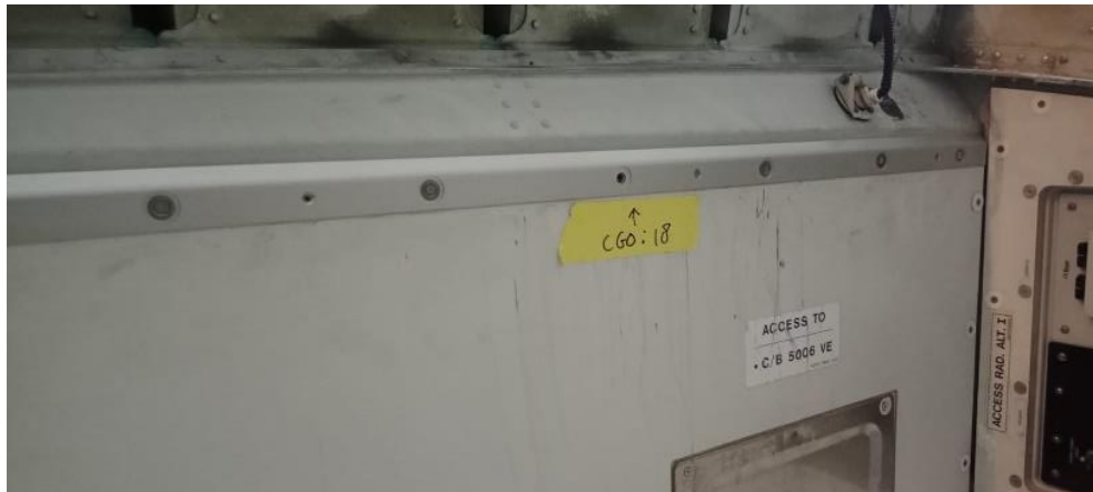
Gambar 4.51 aft cargo ceiling metal lining strip after replacement
