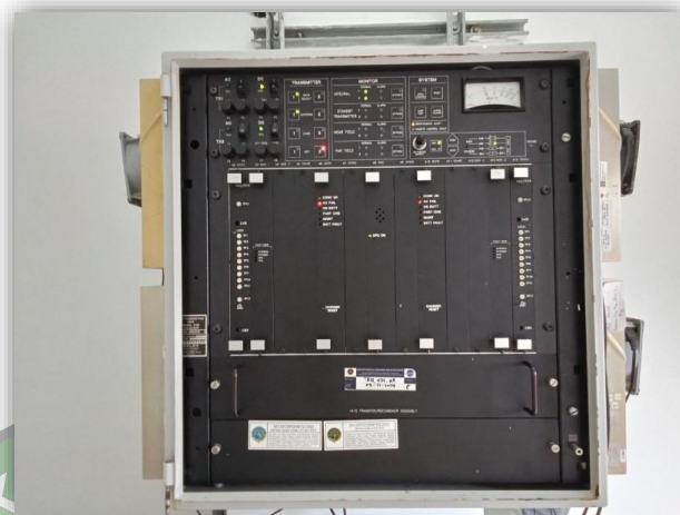
Gambar 3. 18 Peralatan LOCALIZER
