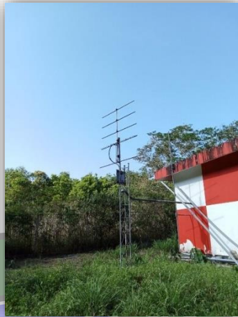
Gambar 3. 19 Antena Middle Marker
