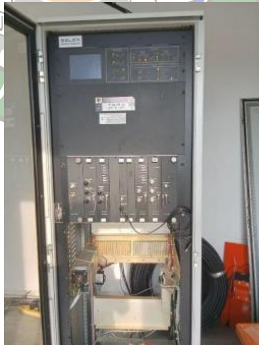
Gambar 3. 20 Peralatan Glide Path
