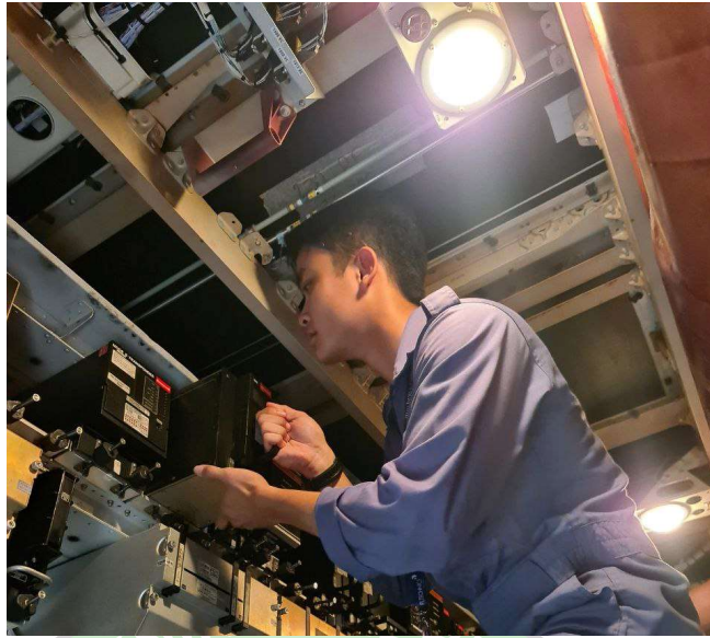
Gambar 4. 16 Pergantian DME Interrogator 1
