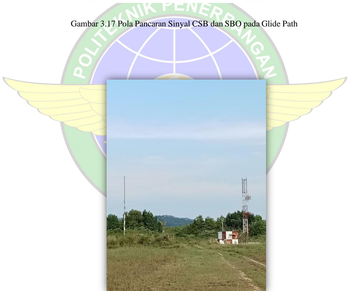
Gambar 3.18 Antenna Glide Path
