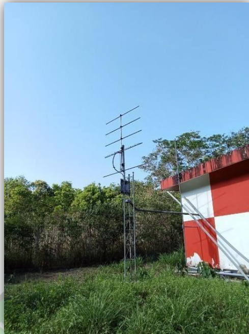
Gambar 3.22 Antenna Middle Marker
