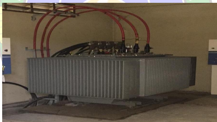
Gambar 4. 6 Transformator Step-Down 1
