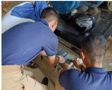
5. Pengecekan panel lampu Flood Light
