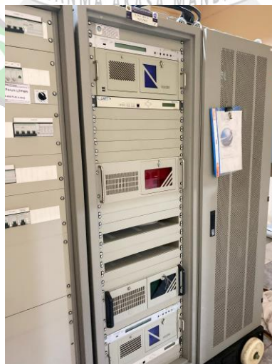
Gambar 3. 16 Rak Radar MSSR
