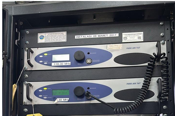
Gambar 3. 15 VHF A/G PAE Secondary TX
