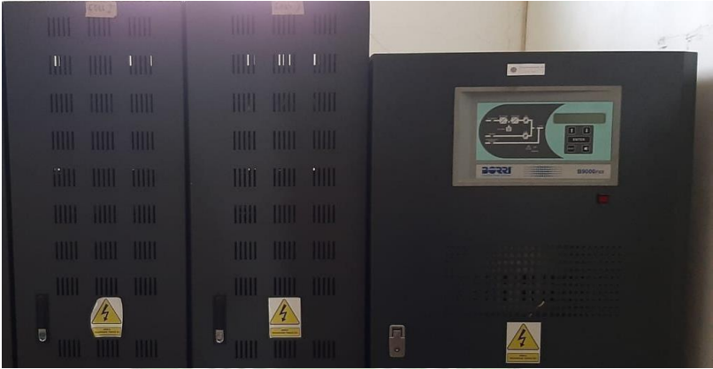
Gambar 2.6 Panel UPS 80 kVA
