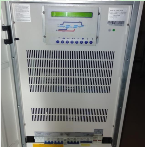
Gambar 2.7 Panel UPS 20 kVA
