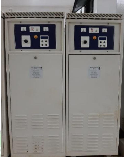
Gambar 2.18 Constant Current Regulator
