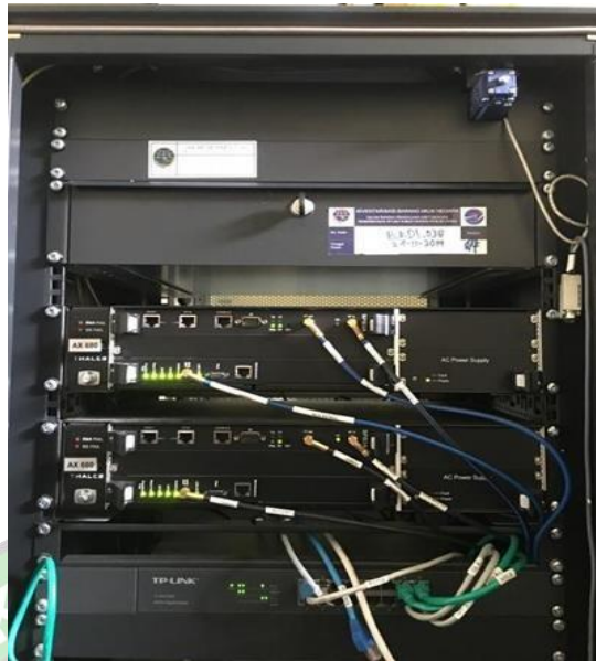
Gambar 3.29 Receiver ground Station ADSB Sumber : Dokumentasi Penulis, 2023
