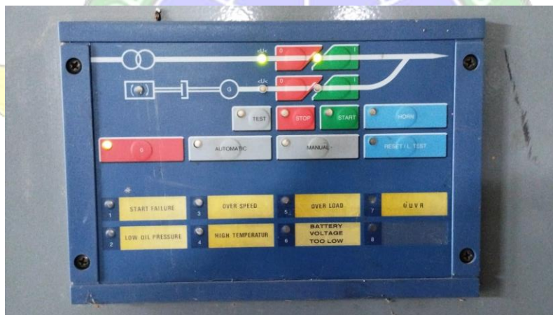
Gambar 4.4 Panel Control Genset PH Bandar Udara Haluoleo Kendari
