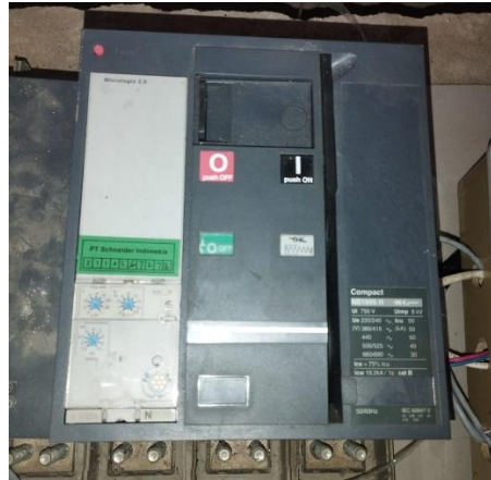
Gambar 3.1 Moulded Case Circuit Breaker (MCCB) motorized Sumber : Dokumentasi Pribadi
