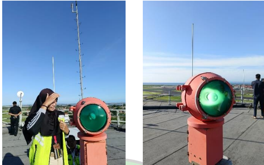
Gambar 2. 33 Rotating Beacon
