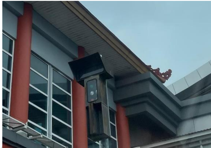
Gambar 2. 35 Aircraft Docking Guidance System
