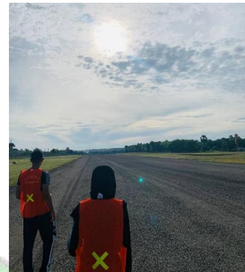
Inspeksi Runway , Apron , Taxiway
