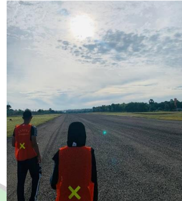
Inspeksi Runway , Apron , Taxiway
