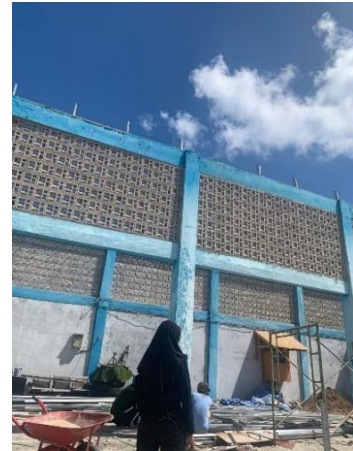
Monitoring renovasi Gedung workshop
