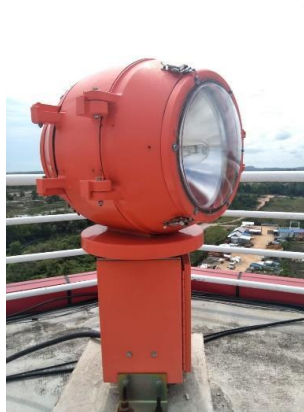
Gambar 2.36 Rotating Beacon
