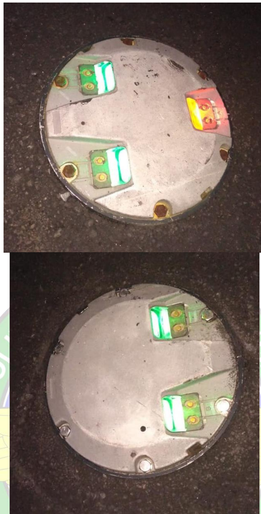
Gambar 2.19 Lampu Threhold
