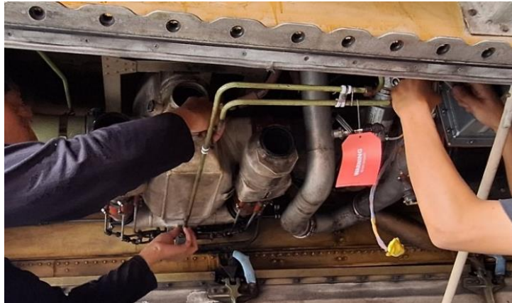
Gambar 4. 20 Remove reheater from the frame assembly (sumber: dokumentasi pribadi)
