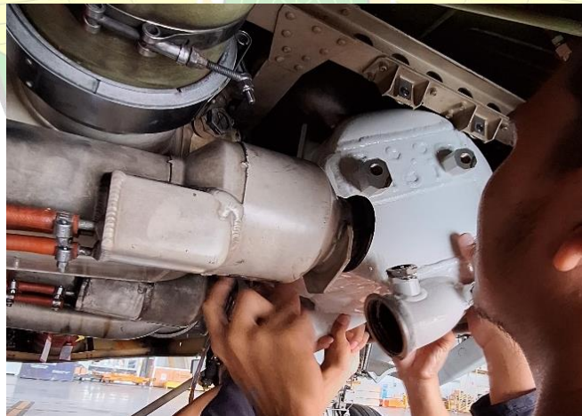
Gambar 4. 21 Install the reheater on the frame assembly (sumber: dokumentasi pribadi)
