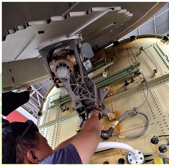
Gambar 4. 18 Weather Radar Receiver/Transmitter Installation (sumber: dokumentasi pribadi)
