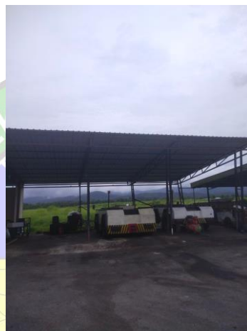
Gambar 3. 3 Equipment Parking Area Sumber: Dokumentasi Penulis
