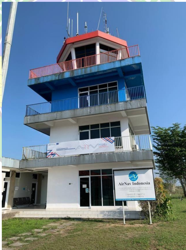
Gambar 2. 2 Tower LPPNPI Unit Tanjung Pandan
