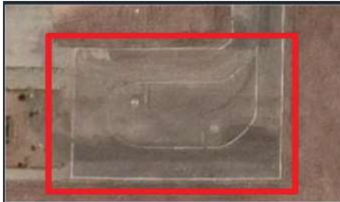
Gambar 4.1 Apron Bandara Tardamu Sumber : Google Earth, 2023
