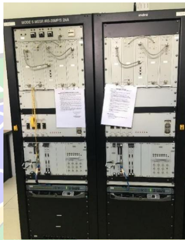
Gambar 3.24 Modul Radar MSSR Mode S INDRA IRS 20/MPS 2NA
