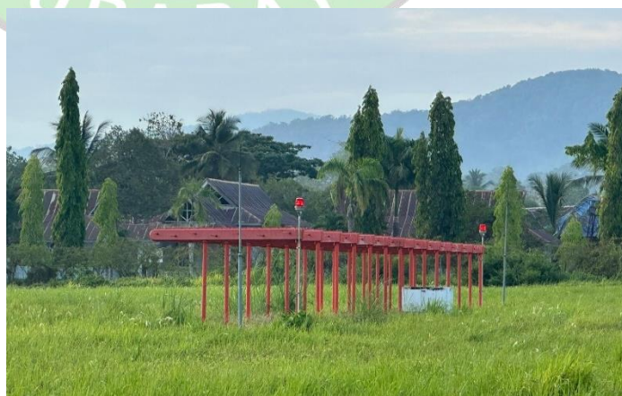
Gambar 3.20 Antenna Localizer
