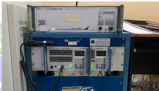
Gambar 3.9 Peralatan VHF A/G EMERGENCY APP
