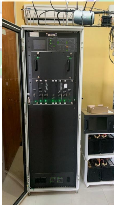
Gambar 3.16 DME collocated DVOR
