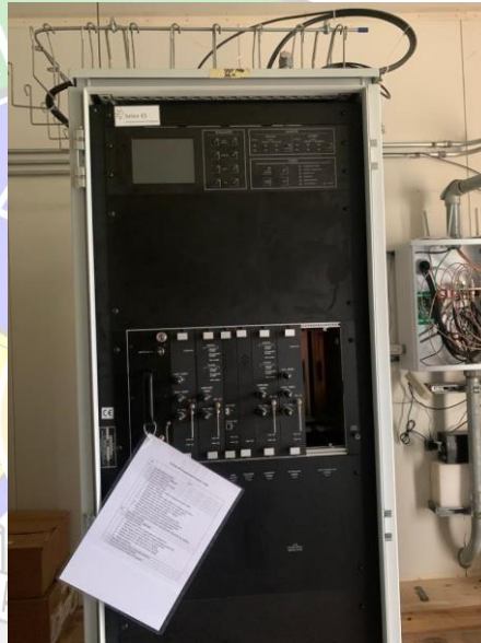
Gambar 3.17 T-DME collocated Glide Path
