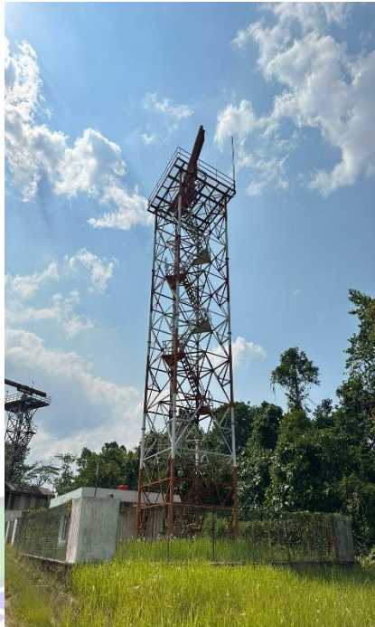
Gambar 3.25 Antena Radar MSSR Mode S
