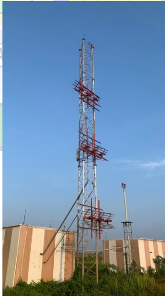
Gambar 3.22 Antenna Glide Path
