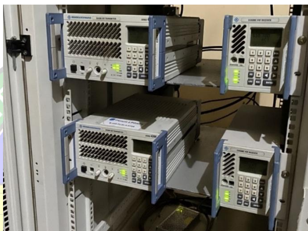
Gambar 3. 4 Transmitter dan Receiver VHF A/G ER TWR
