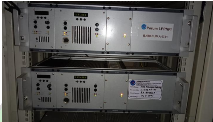
Gambar 3. 5 Transmitter dan Receiver VHF A/G ( Secondary ) TWR
