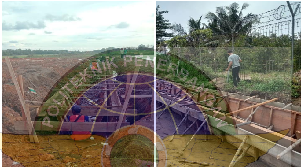
Gambar 4. 20 Bekisting Dinding
